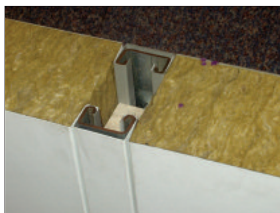
Figure 17: Insulated core panels – internal
