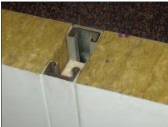
Figure 16: Insulated core panels – internal panel
